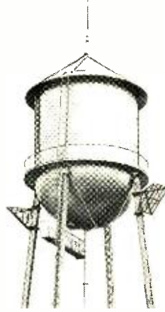
Reflectors on tank at Grande Ecaille.
